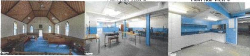
Main Hall View 5
